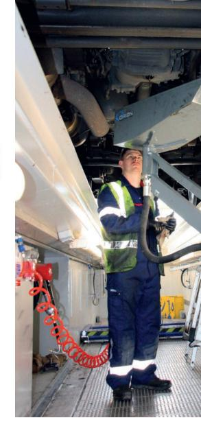
will often provide a very good clue as to why a unit has failed. All of the used oil - whether it be engine, gearbox, axle or transmission - goes into the same tank. The tank will need emptying every two or three months. It is discharged by gravity into a collection tanker." (Draining manifold shown top right.)
